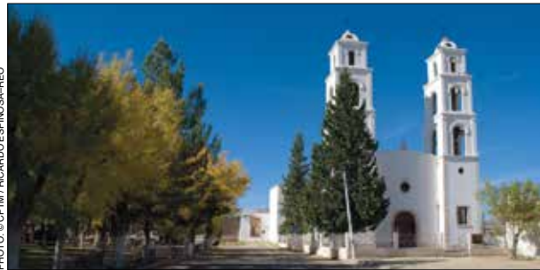
Parish Church of San Antonio de Padua, Casas Grandes.
